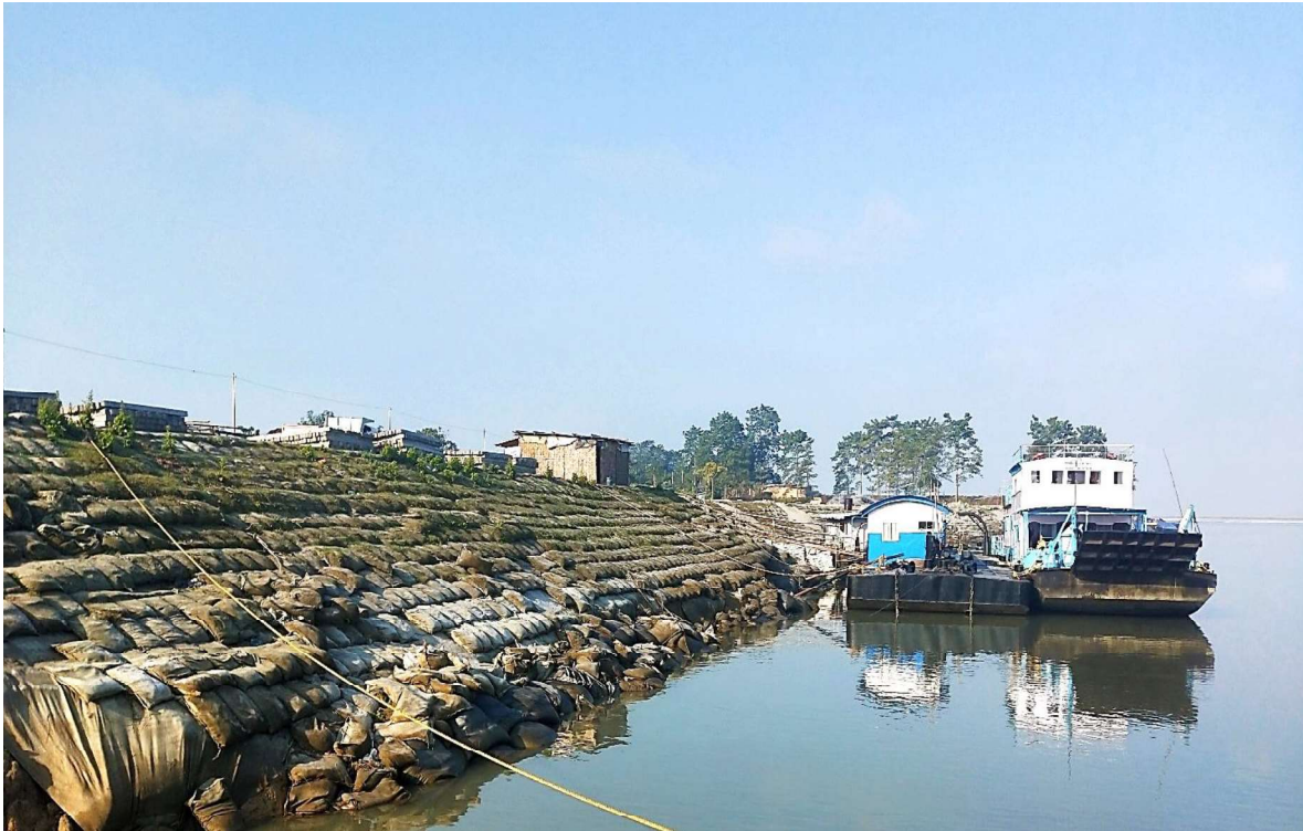
Figure 8-15 Placement of Geo-bags at the river bank - Neamati
